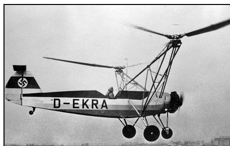
3. ábra. Focke-Wulf Fw 61 helikopter (forrás: http://en.wikipedia.org/wiki/FW-61 )
