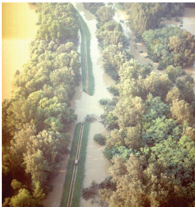
Figure 9 | Dike breach at Surány (Danube right bank) 09 August 1991 Source: ABKSZ
