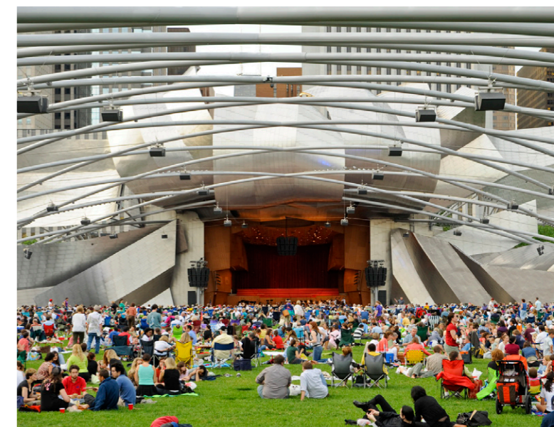
Figure 3: A big advantage of the design concept in the Millennium Park at the Jay Pritzker pavilion is bringing the sources of sound closer to the auditorium, which enables lower volume to make the performance enjoyable, making it less disturbing for the surrounding residential areas [34]. (Designer: Frank O. Gehry, 2004., USA) https://www.archdaily.com/892320/the-jay-pritzker-pavilion-gehry-partners , (2020. 07. 20.)
