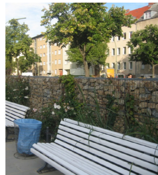
Figure 2 a, b: Audio islands and gabion noise screens at Nauener Platz in Berlin, where soundscape design decisions were based on monitoring the noise levels on site [29]. (Researcher and designer: Prof. Dr. Brigitte Schulle-Fortkamp, 2011-2012, Germany) https://www.researchgate.net/publication/306085310_WHEN_SOUNDSCAPE_MEETS_ARCHITECTURE , https://sonicagents.wordpress.com/2013/01/04/a-soundscape-re-modeled/#more-264 , (2020. 04. 30.)
