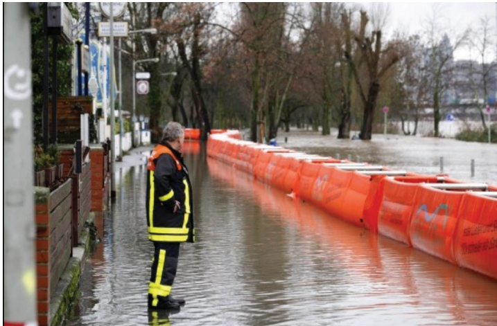
Figure 8. Rapid-deployment mobile dykes. (Made by Dapd, [40])
