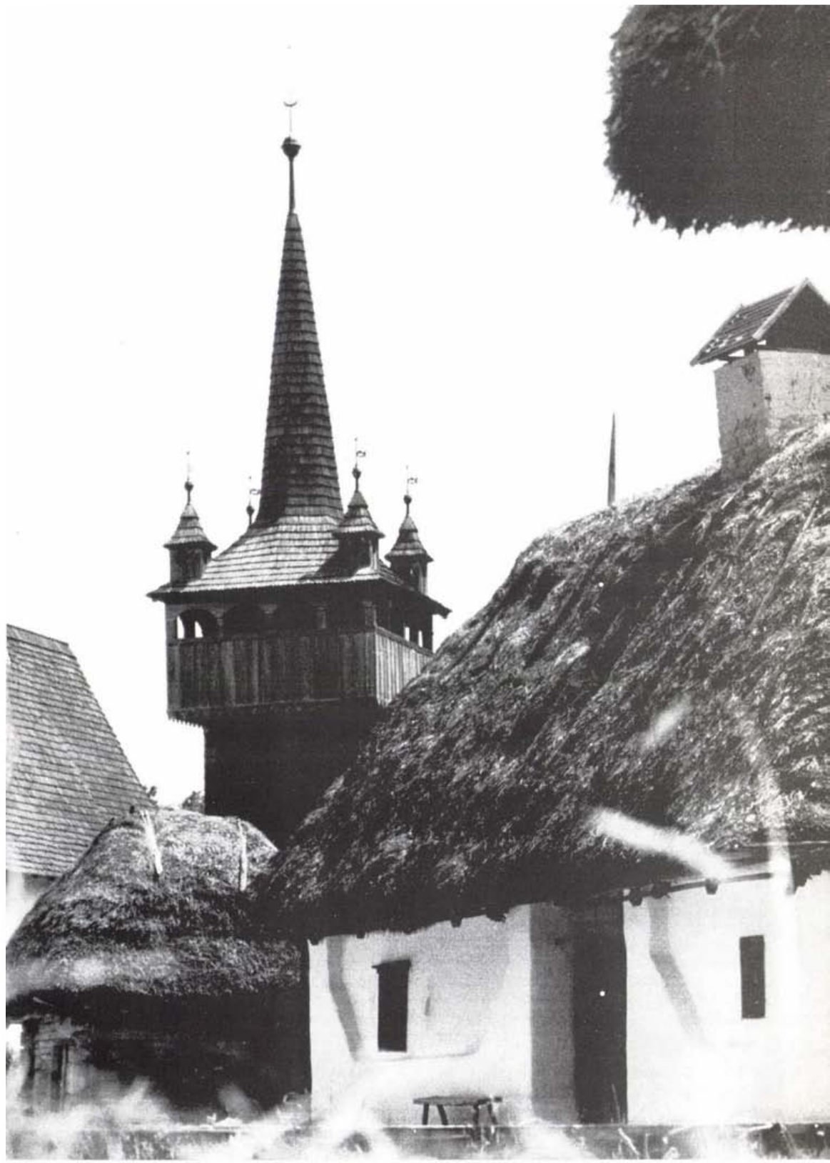
St. Martin's Church, Krasno Selo, Bulgaria. The church is a fine example of the traditional wooden architecture of the Balkans. The photograph was taken in 1954 by the author.
