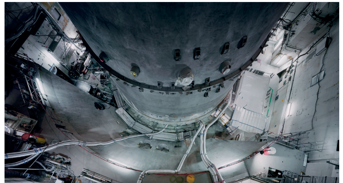
Reactor Pressure Vessel Phase Out, AKW Würgassen, Biberach, 2009 Chromogenic print, 171,0×305,0 cm © THOMAS STRUTH
