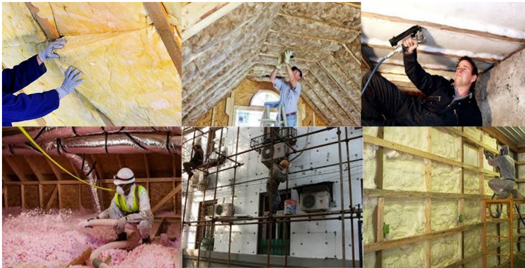
Figure 4. Insulations applied to the interior and exterior building envelope.
