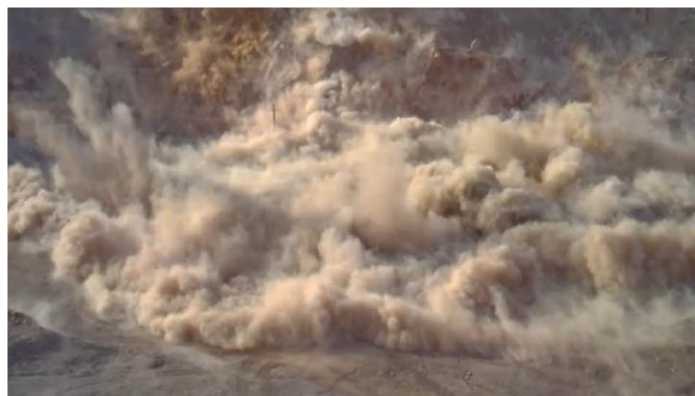
Figure 1. Blowing dust after blasting
