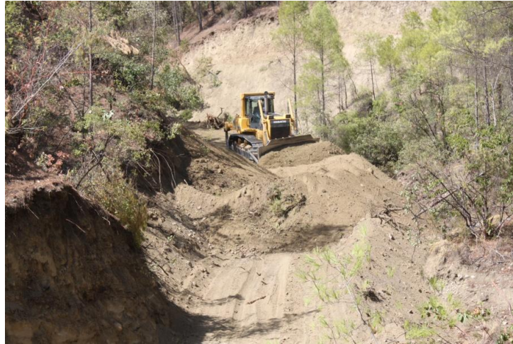
Figure 6. The fill with excavated material of stream bed
