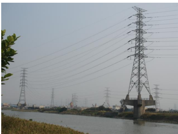
Figure 26. No. 10 and No. 12 towers
