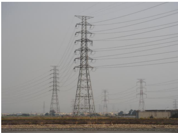
Figure 8. No. 7 tower (the second from the left)
