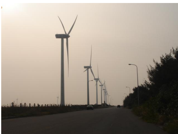
Figure 14. No. 21 wind turbine
