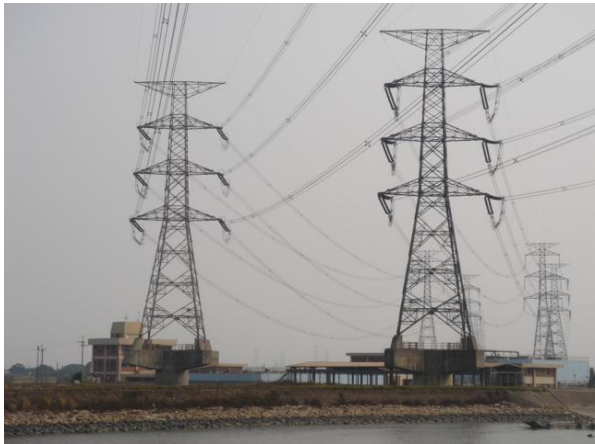
Figure 4. No. 26 tower (right side)
