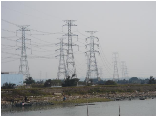
Figure 6. No. 31 tower (the second from the left)
