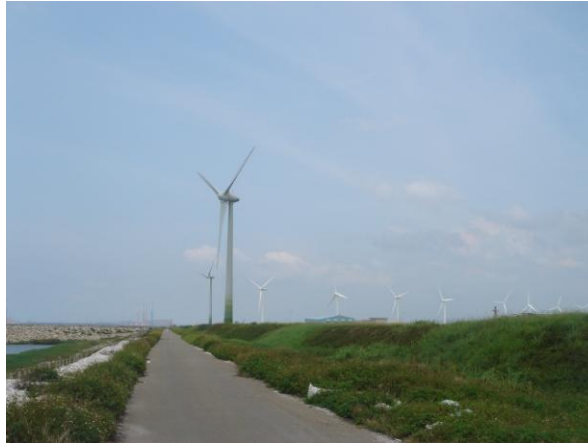
Figure 3. Wind power generation facilities in coastal areas in Chang Bin coastline
