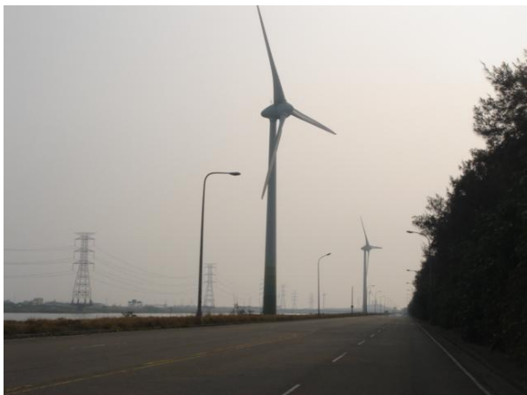
Figure 12. No. 34 wind turbine
