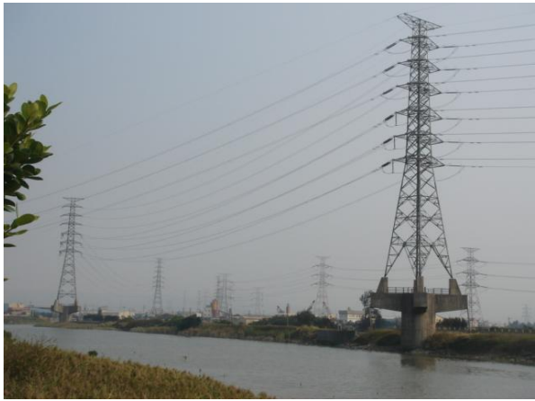
Figure 28. No. 10 and No. 12 towers
