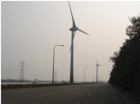
Figure 18. No. 34 wind turbine
