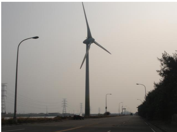
Figure 20. No. 33 wind turbine
