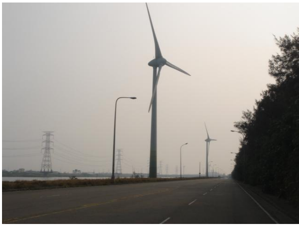
Figure 10. No. 34 wind turbine
