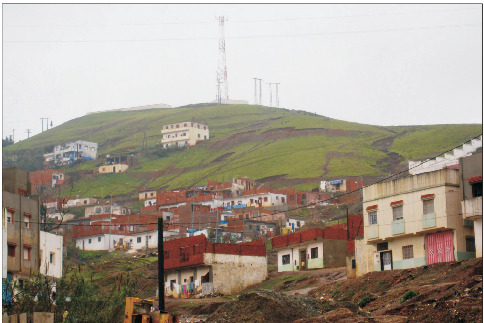
Photo 2. Areas prone to landslides in Korrat Sbae. Source: Faculty of Sciences, Tétouan, 2012.
