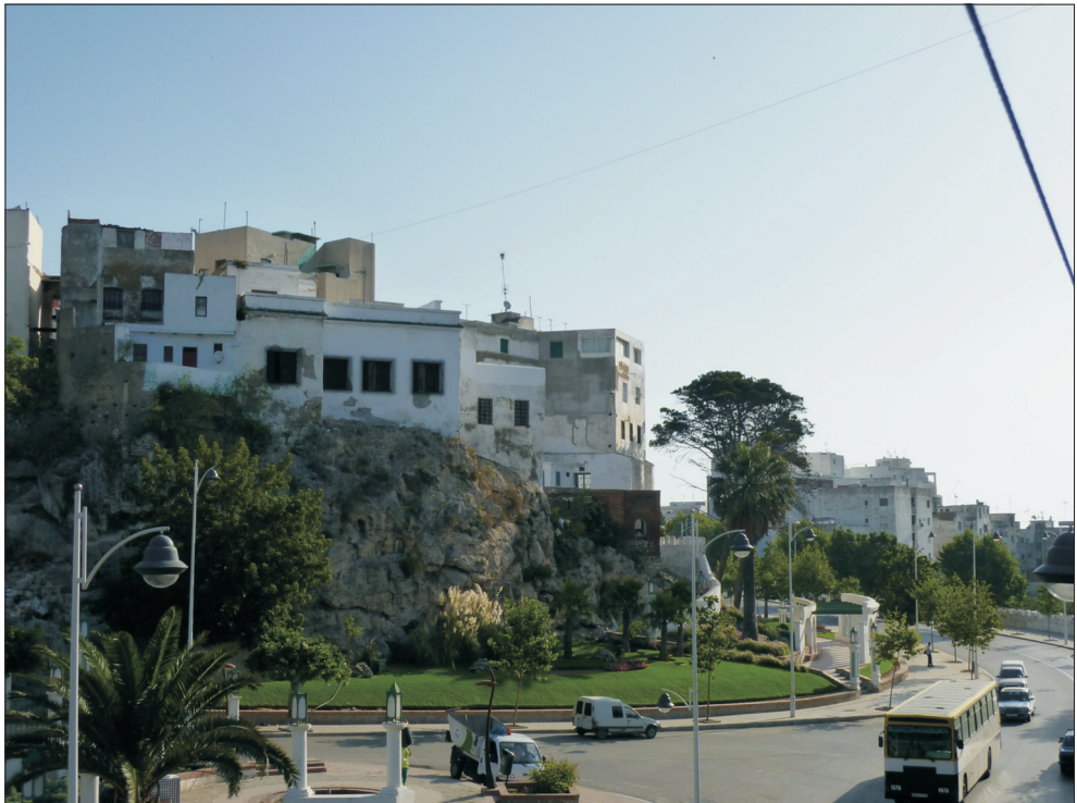
Photo 5. Houses built on travertines in the downtown. Source: Faculty of Sciences, Tétouan, 2013.
