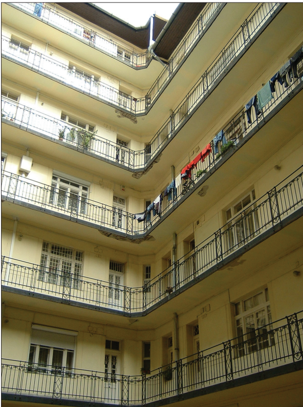
Photo 4. Hanging corridors in the inner courtyard of a tenement block built at the turn of the 20th century. Source: RÉV8 Urban Development Company
