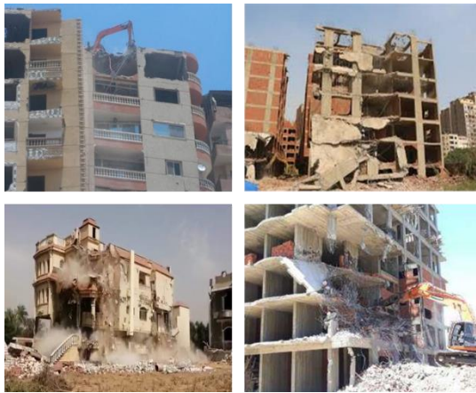
Figure 2. Examples of Demolishing Buildings [25]
