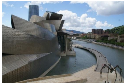
Fig. 3 The curving surface of the iconic Guggenheim Museum in Bilbao (Frank O. Gehry)
