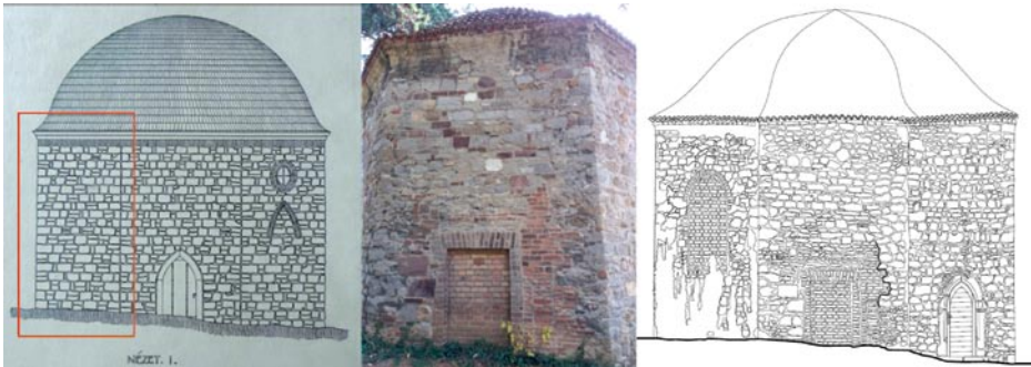
Figure 6. Drawing of the North-western façade by Sinogli, supervised by Foerk in 1917 and the current status of the façade (MMA MÉM MDK Plan collection 13213/a, photo and survey drawing of the authors, 2015)
