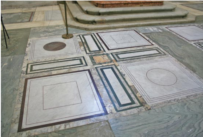
Figure 4. Early Christian floor reconstructed by means of the results of true-to-form survey on the Santo Rotondo Church in Rome
