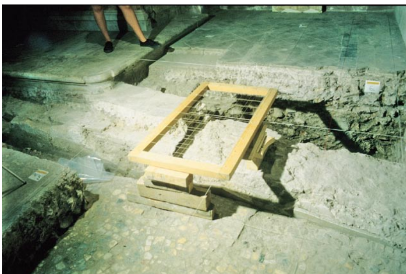
Figure 1. Tools of true-to-form survey: a cord-net independent of the building and a skeleton frame of square grade
