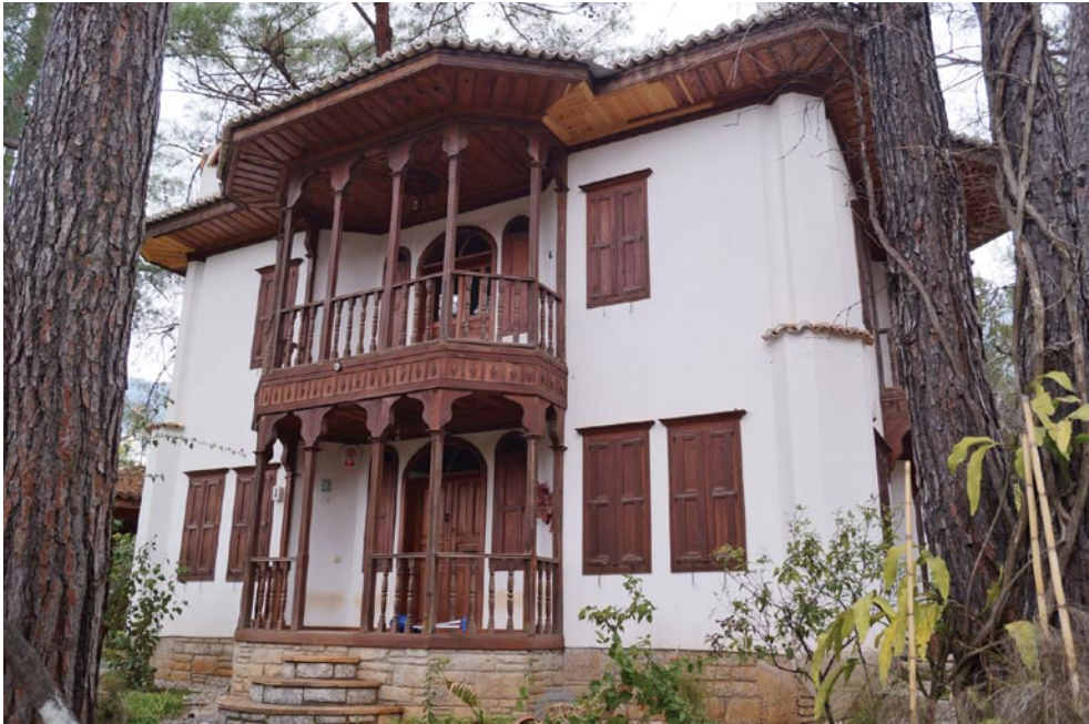
Figure 18. Sevgi Öncü House (Source: Author).
