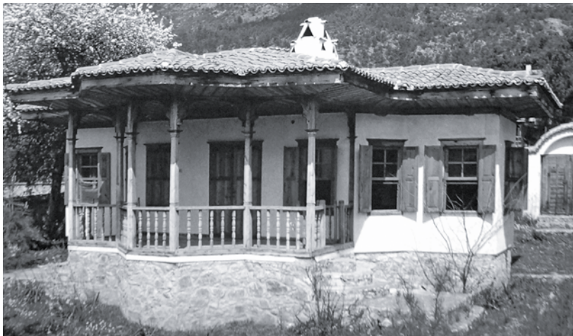
Figure 13. Minu İnkaya House (Çakırhan 2005: 63).
