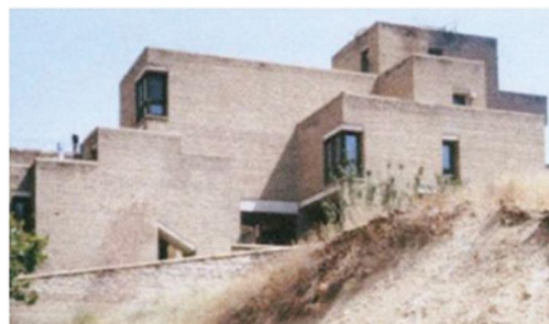
Figure 9 Alizade's attempt in paying attention to traditional aspects like privacy (few small windows in street side).
