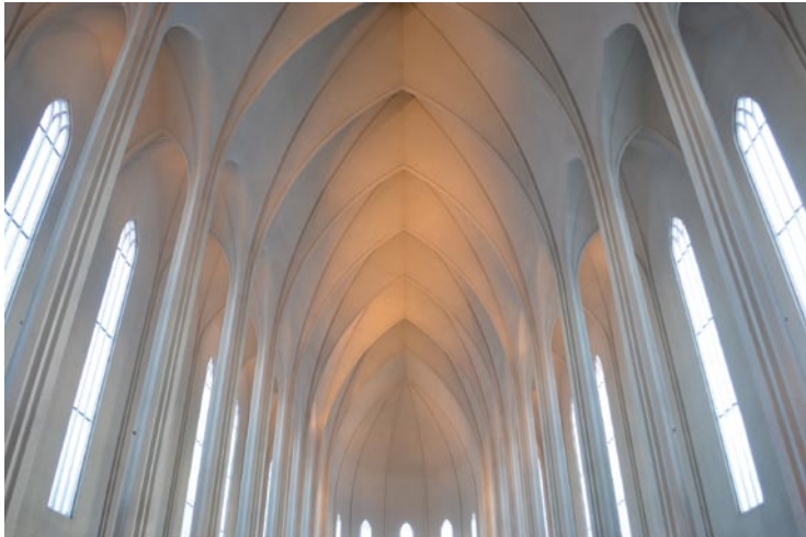
Figure 10. The vaulting of the nave.
