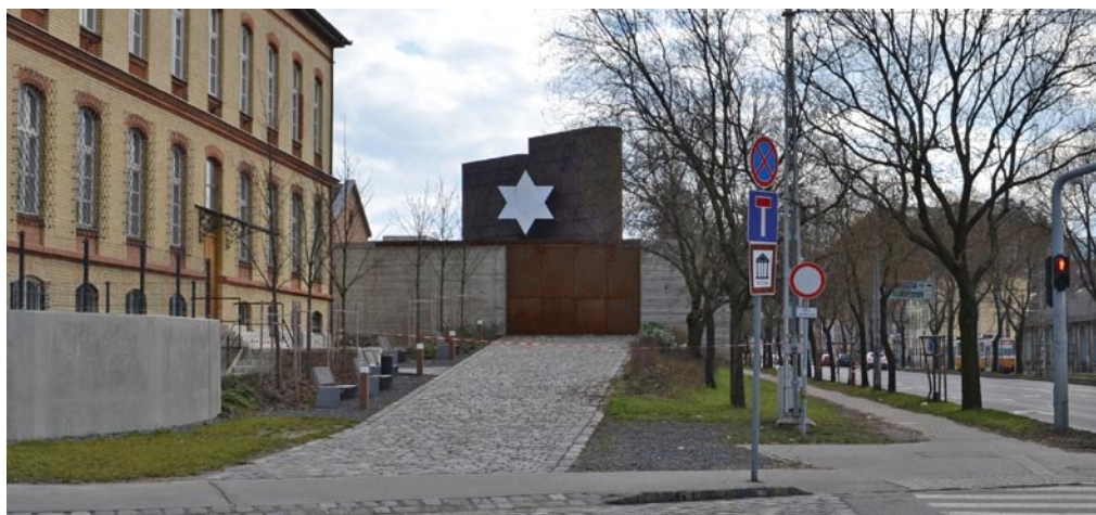
Figure 2. View from Salgótarjáni Street
