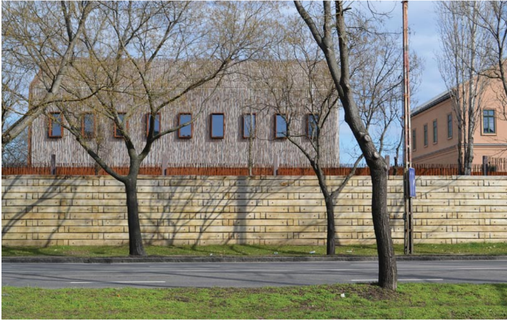
Figure 4. Ancillary building from the side of Fiumei Road
