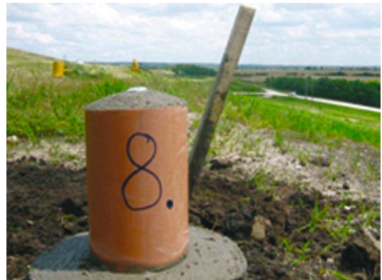
Figure 5. Settlement measuring point.
