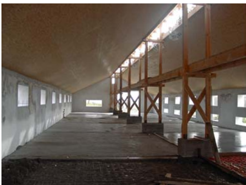
Figure 11-13 Application of ridge ventilators in a bio hen house and a multifunctional storing building (architects: Dr. Gábor Reischl, Zoltán Laczó)
