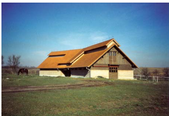
Figure 31 Ridge ventilators ensuring natural ventilation in a stable in Mende (architect: Dr. Gábor Reischl)
