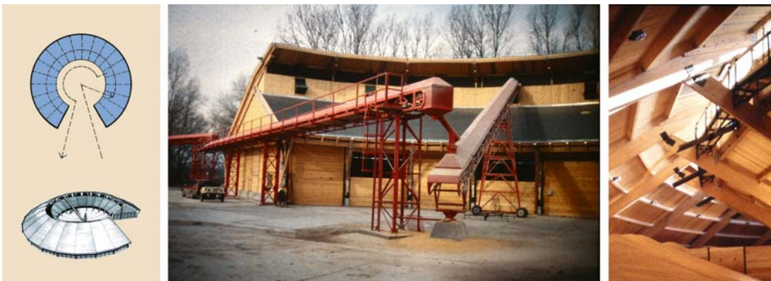
Figure 18-20 Operational principle of the with 6000 tons grain crops storing building in Balatonfenyves and the feeding, ventilating and lighting opening from outside and inside (architect: Dr. G abor Reischl)
