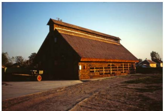
Figure 11-13 Application of ridge ventilators in a bio hen house and a multifunctional storing building (architects: Dr. Gábor Reischl, Zoltán Laczó)
